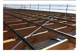
DriSpace VENT System is designed to support the mitigation of mould, excessive moisture build-up, and condensation in roof cavities when the system is installed and maintained in accordance with DriSpace's guidelines.
