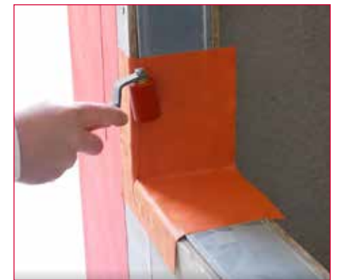
Fig.06: Use roller to ensure proper adhesion of Wraptite Corners to substrate.
