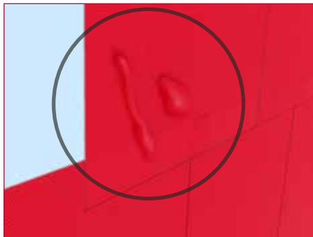
Fig.03: 'Bubbles' caused by insufficient pressure when installing Wraptite.
